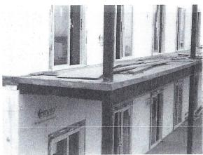
• The second floor unit walls are ICF and are attached to the first floor with poured concrete and locked into place with the Hambro bar joists.
