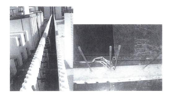
• The Hambro System forms the second floor and consists of a specialized steel bar joist beam that is attached to and sits atop the solid concrete ICF wall.
