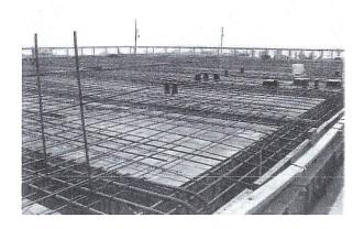
• The platform gives rise to the concrete walkways and balconies that are also reinforced with steel rebar and are totally supported by steel reinforced beams in a cantilevered system.
